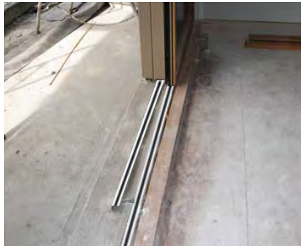
Filling in Concrete Base
