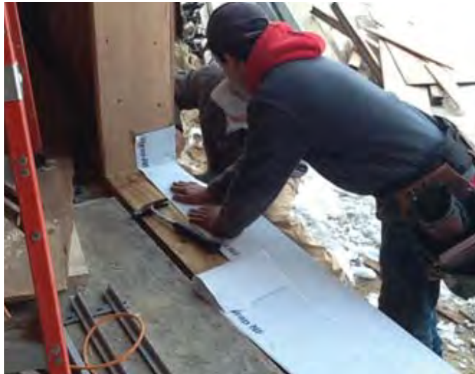
Flexible Sill Pan Installation
