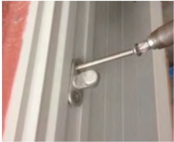
Final Hardware Install
