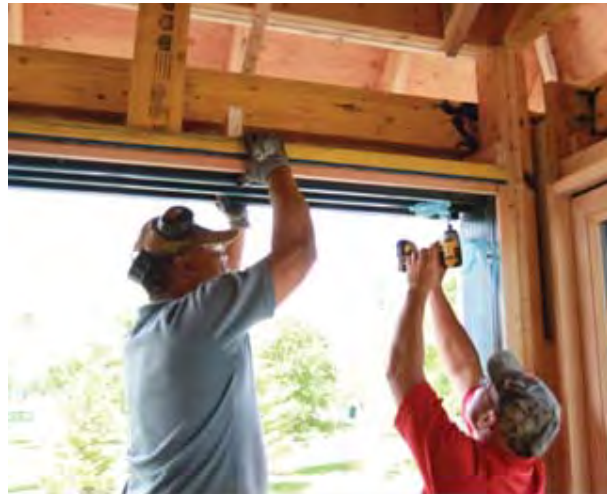
Head Track Installation
