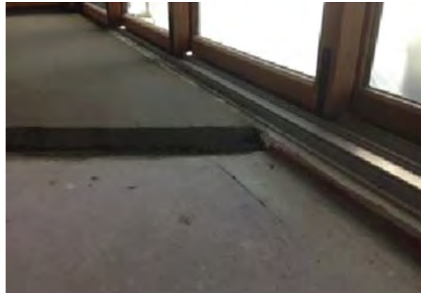
Filling in Concrete Base
