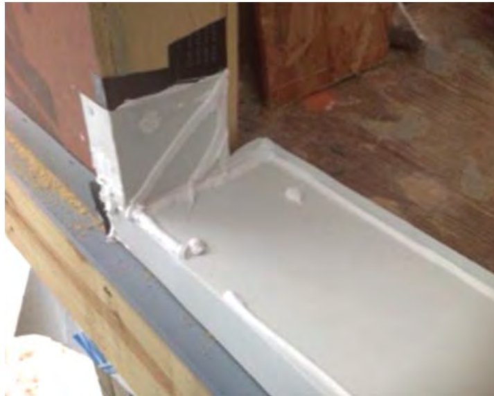
Rigid Sill Pan Installation
