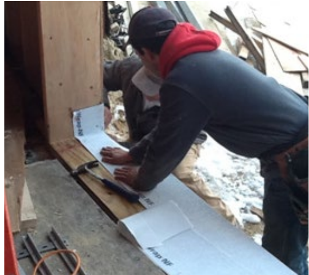
Flexible Sill Pan Installation
