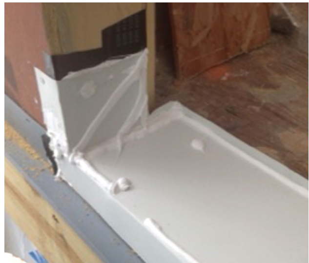
Rigid Sill Pan Installation
