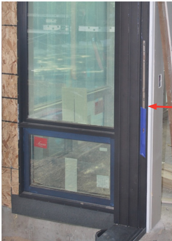
Interior track with strike plate.
