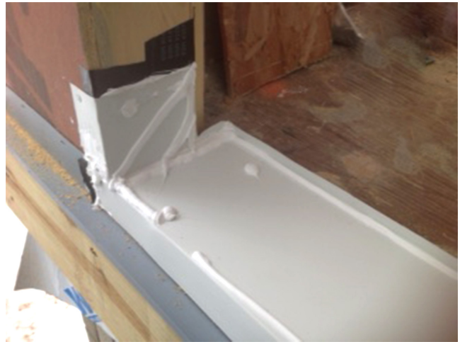
Rigid Sill Pan Installation
