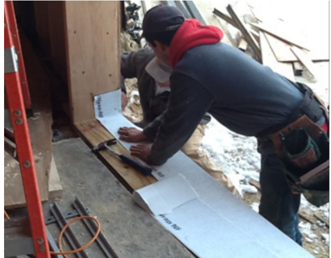
Flexible Sill Pan Installation
