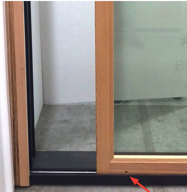
WHEEL ADJUSTMENT ACCESS HOLES
